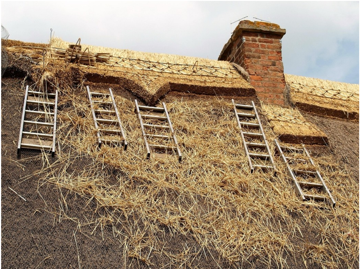
Reparatur eines alten Reetdachhauses, August 2017, © Sue Rickhuss, public domain
